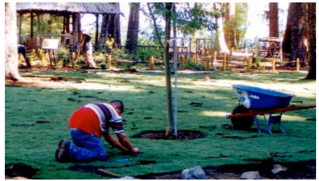
Laying the Sod
